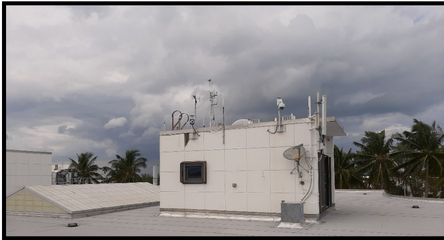
Figure 5.2 South facing in
