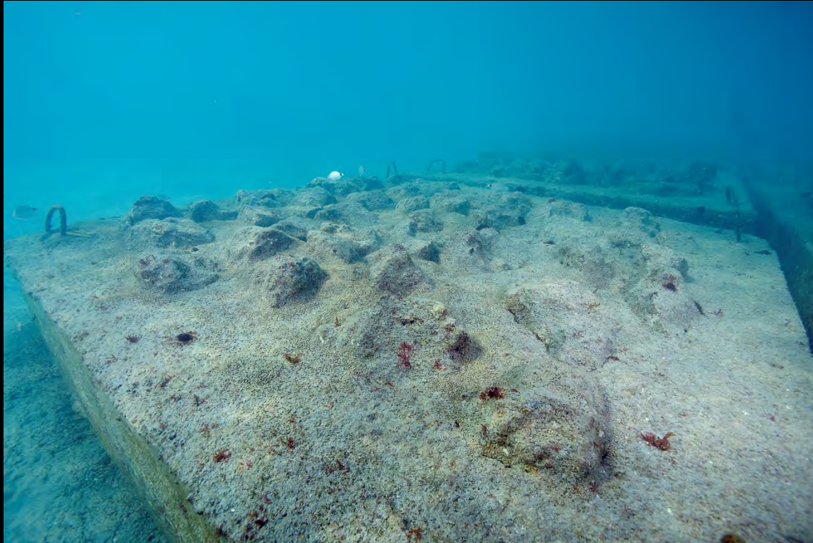
Singer Island concrete module
