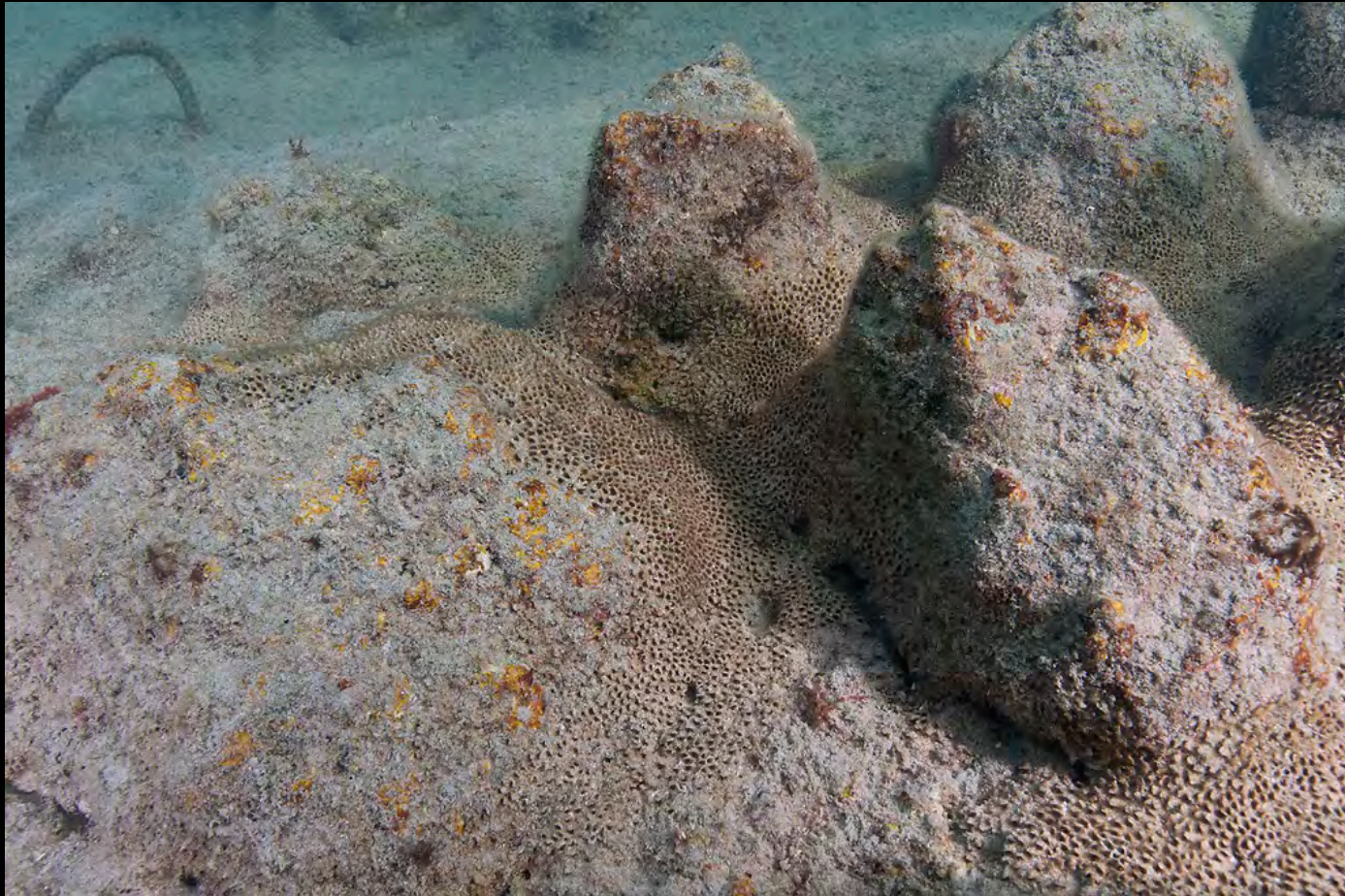
Singer Island concrete module
