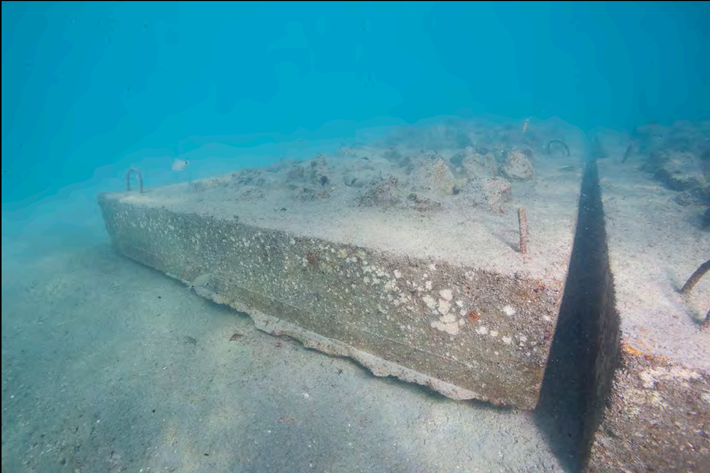
Singer Island concrete module
